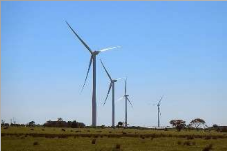
Mt. Mercer wind farm (currently under construction)
